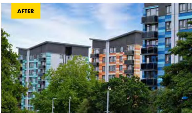
RECLADDING CHARLEMONT FARM ESTATE, UK.
